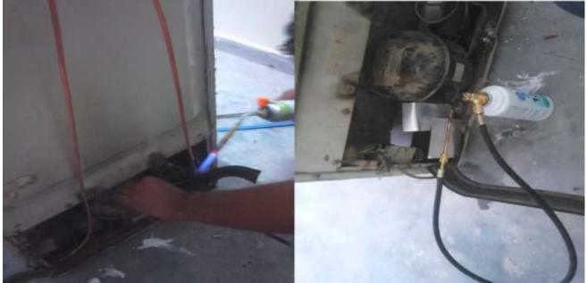
Fig 1.4: Welding of copper tubes and gas filling by cylinder.
